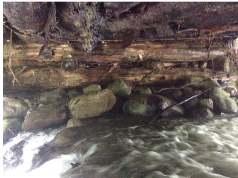
Right Bank Abutment when facing downstream
